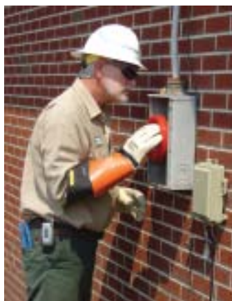
Service Technician Ken Winslow installs a collar for disconnecting service at a meter base.
